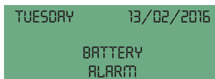
Battery fault indication
